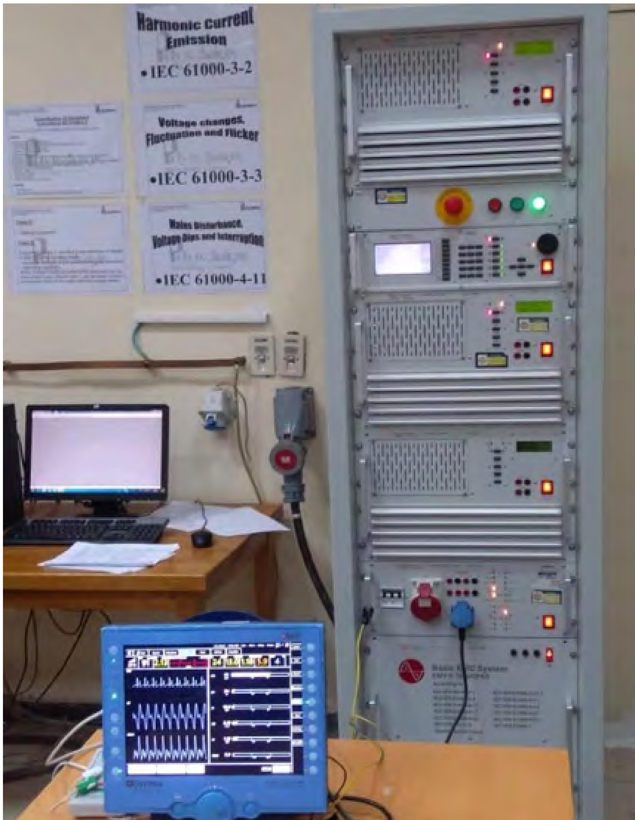
Fig. 27: Harmonic Current Emission Test Setup
